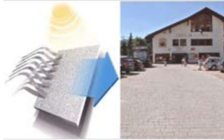
Fig. 10: Concrete paving panels with photo catalytic air purifying properties used as a design element in a car park.
