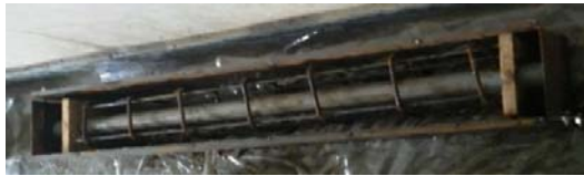
Fig: 2 Casting of beam specimen
