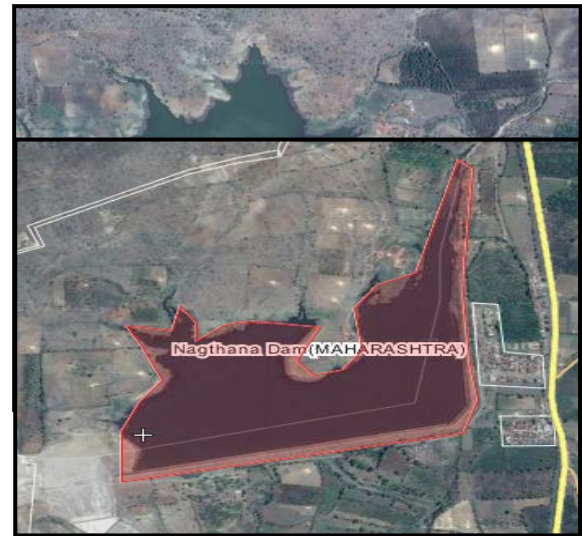
Fig. 4 Satellite View of Nagthana Dam
