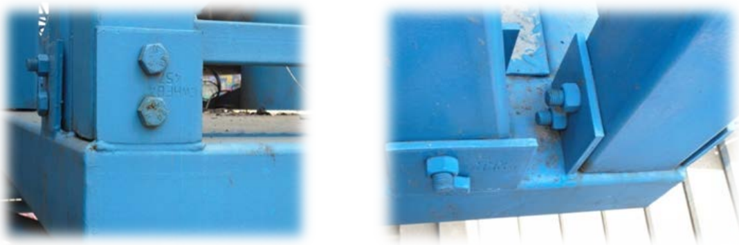
Fig 08: Typical pinned connection we found at our site investigation.
