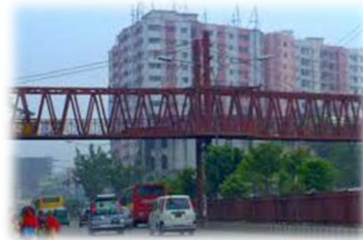
Fig 07: Typical view of foot over bridge.
