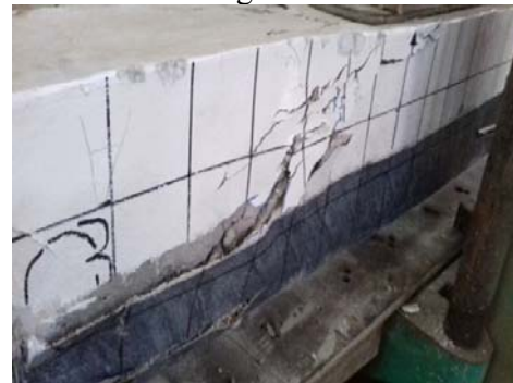
Photo4. Girder C3 - Strengthening Length = L
