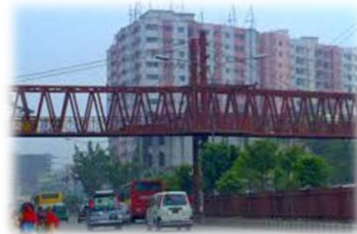
Fig 07: Typical view of foot over bridge.
