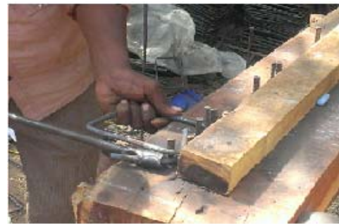
Fig.1 Manually stirrup making process
