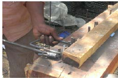
Fig.1 Manually stirrup making process
